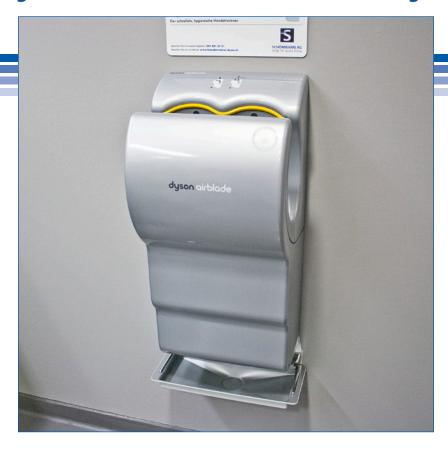
SCHÖNMANN AG produces drip trays for the Dyson Airblade hand dryer so that the water removed from the hands during drying does not fall on the floor.
